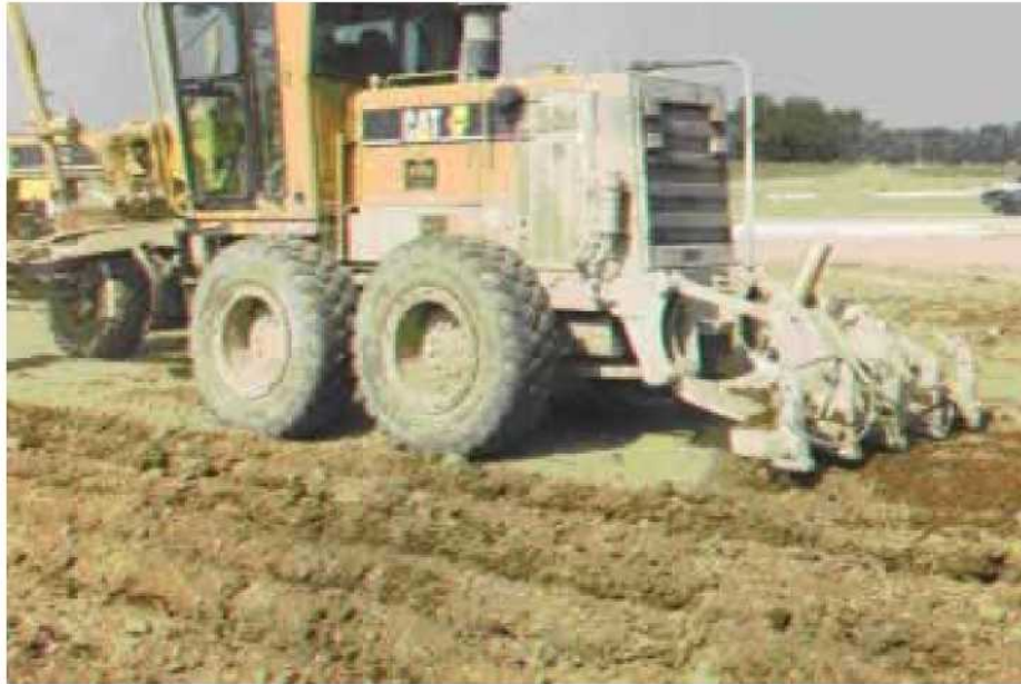
Figure 8: Scarification before lime application
