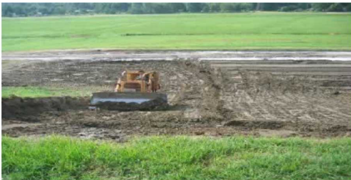
Figure 24: Returning treated soils from mixing area to embankment
