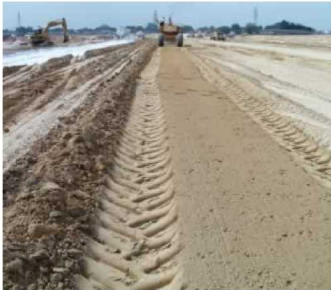
Figure 16: Mixing and pulverization
