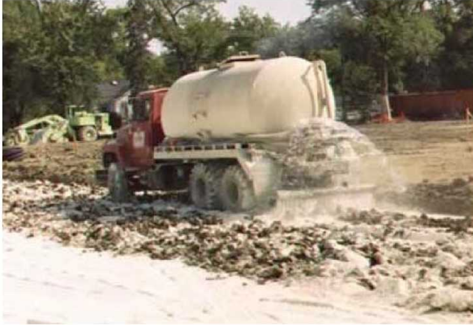
Figure 13: Adding water after dry lime application 5
