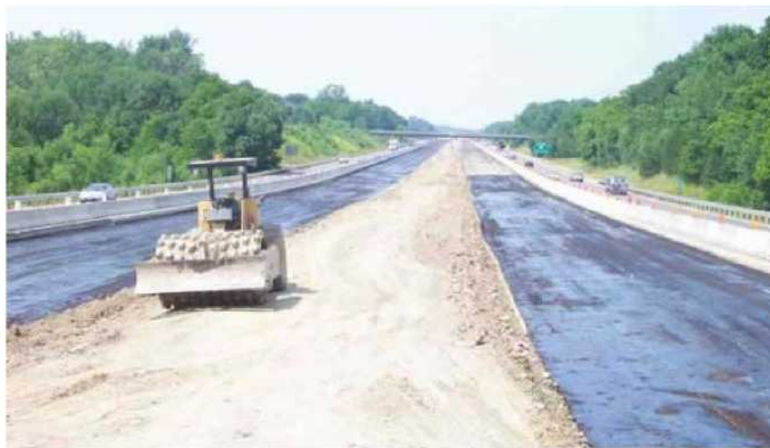
Figure 19: Prime coat emulsion for curing
