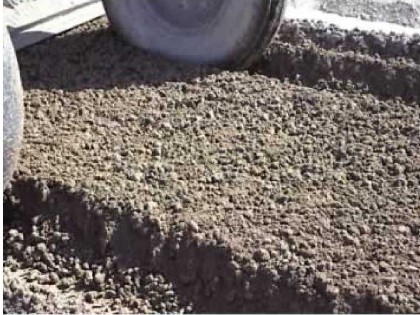
Figure 4: Lime flocculating clay
