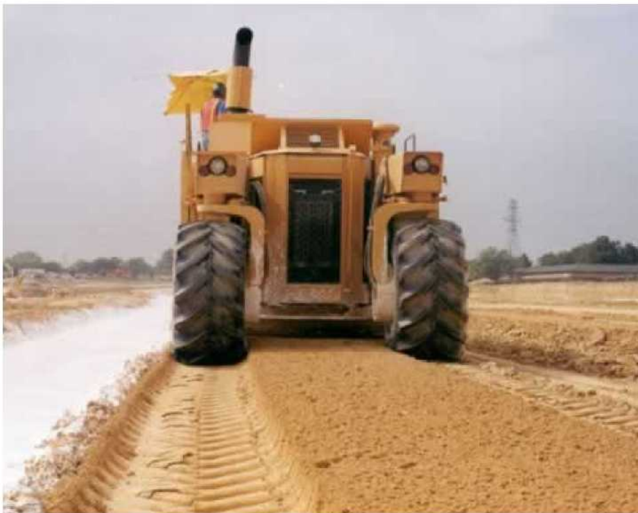
Figure 14: Rotary mixer used for initial mixing
