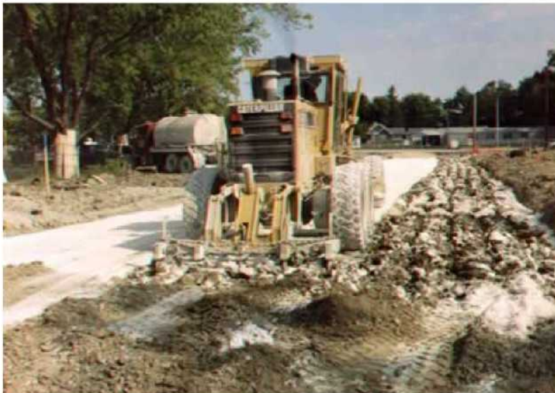
Figure 12: Scarification after lime spreading
