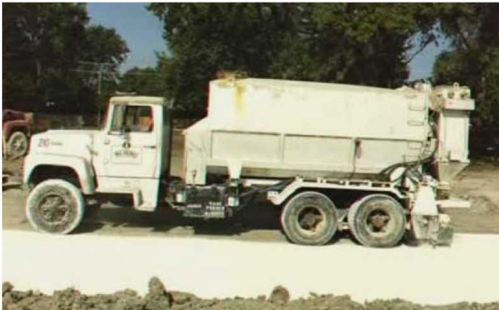
Figure 10: Dry lime application with mechanical spreader 4
