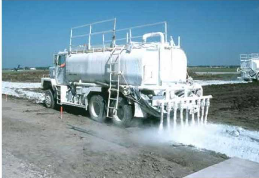
Figure 11: Example of lime slurry application
