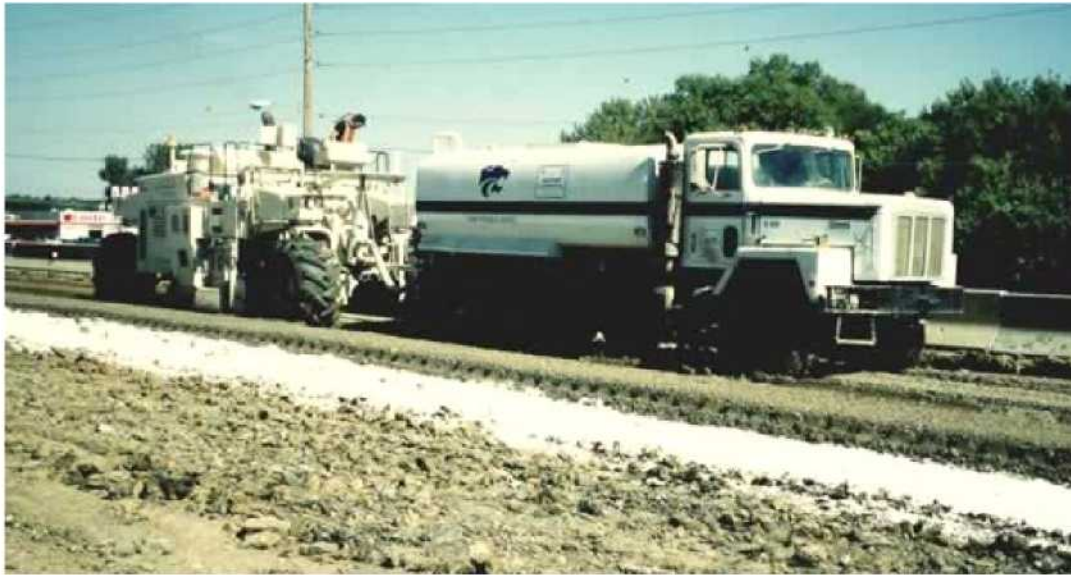
Figure 15: Rotary mixer with water truck attached
