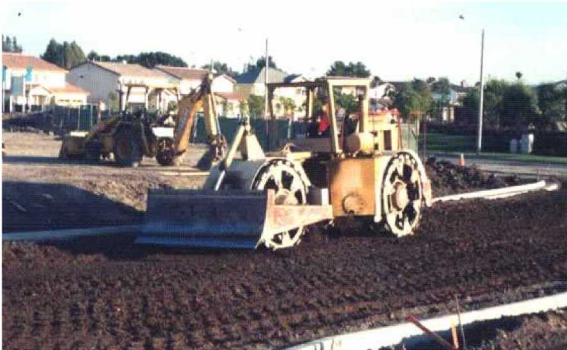
Figure 22: Compacting lime stabilized soil for base of street in housing subdivision
