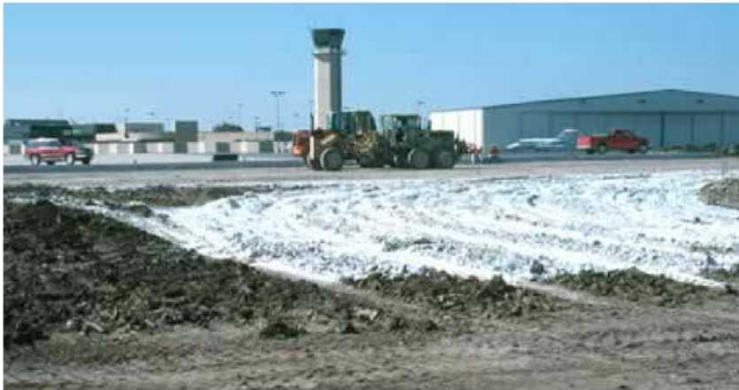
Figure 21: Lime stabilization project at an airport
